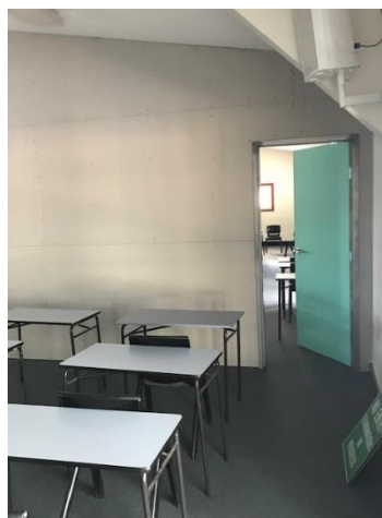
Two temporary walls were built in the Houlston Centre to break the large exam space up into three smaller spaces which meets the Department of Education requirements for COVID-19
