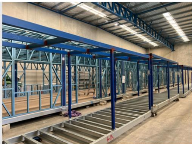
Deck/walkway facing bottom
